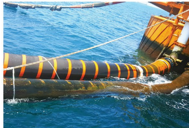
首管 First offbuoy hose
